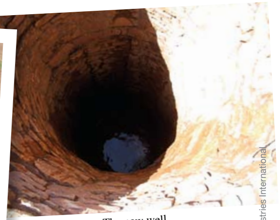
The new well.
